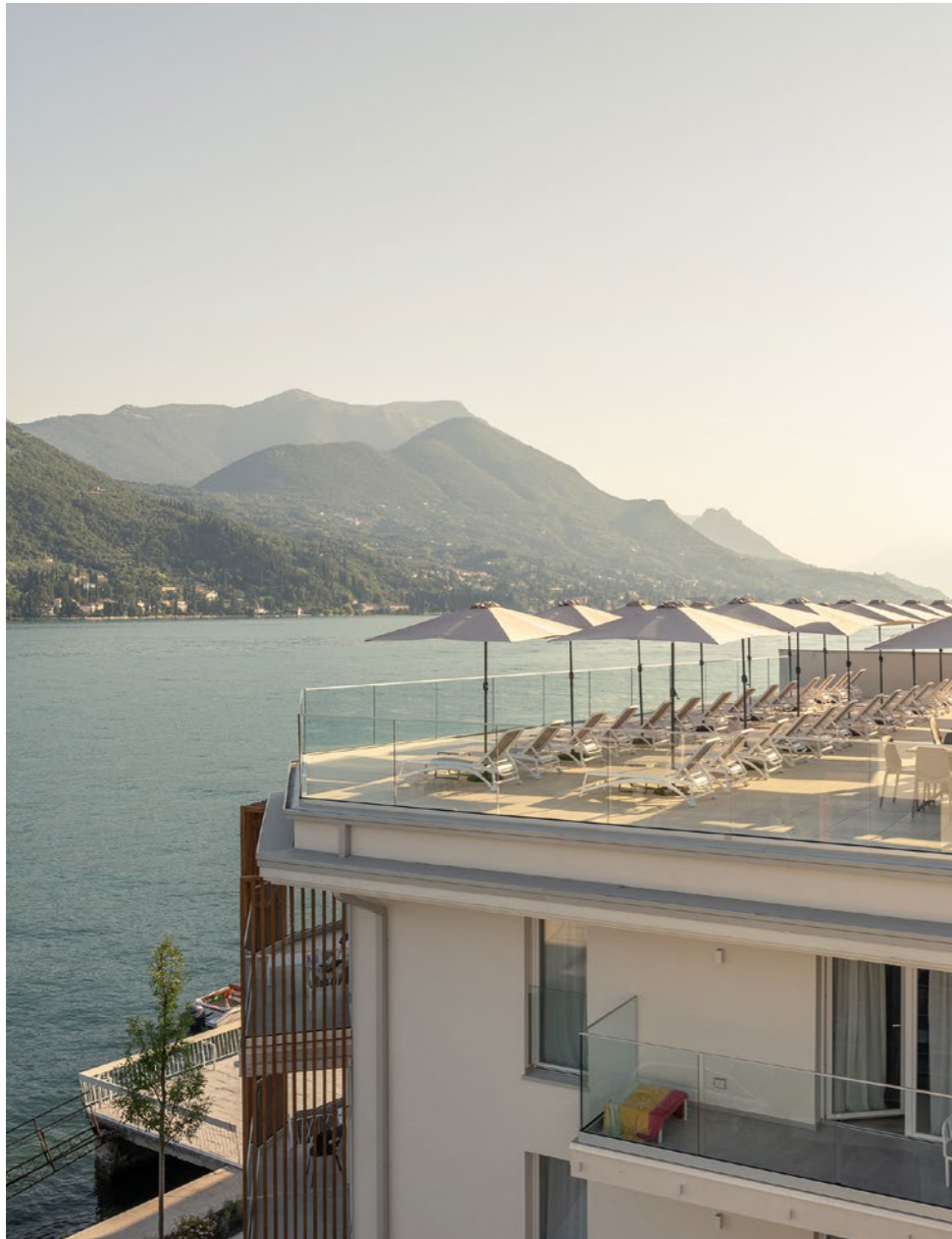
AH Porticcioli Boutique Apartments Resort San Felice del Benaco - Italy Project: Hotel Products: Atlantico, Pop
